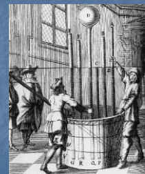
Torricelli's barometer experiment
